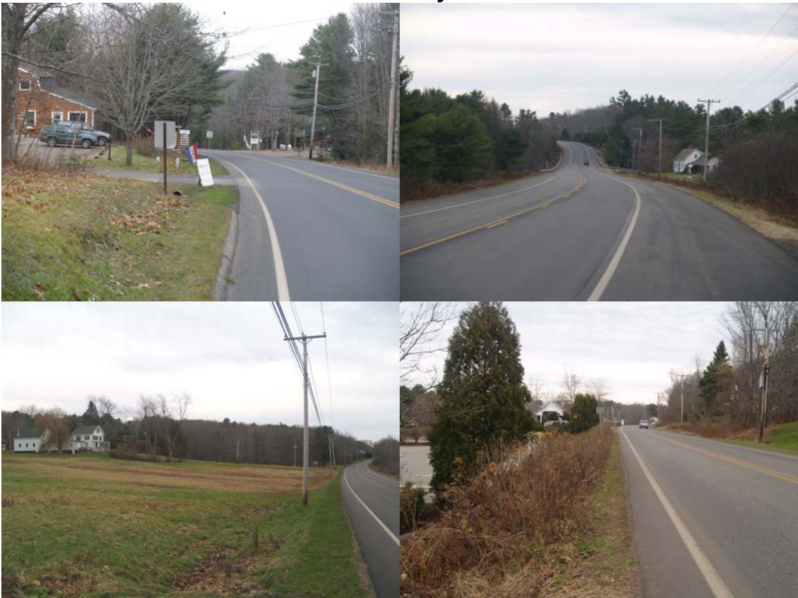
Figure 13 Variable Width Shoulders on Route 27 North of Boothbay Common
